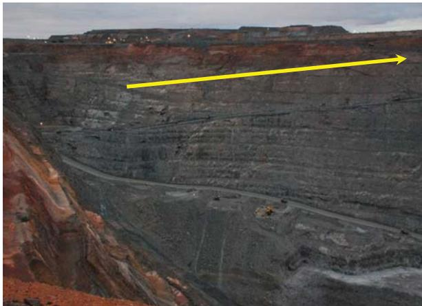
*Figure 3. KCGM Mine Haul Road. Tiny Objects on Haul Road are 240-Ton Trucks. A Truck Breakdown on the Haul Road Can Shut Down Much of a Mine.*
